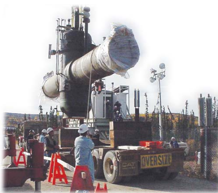
TAPS workers replace a 48-inch gate valve north of Coldfoot in 2002.
