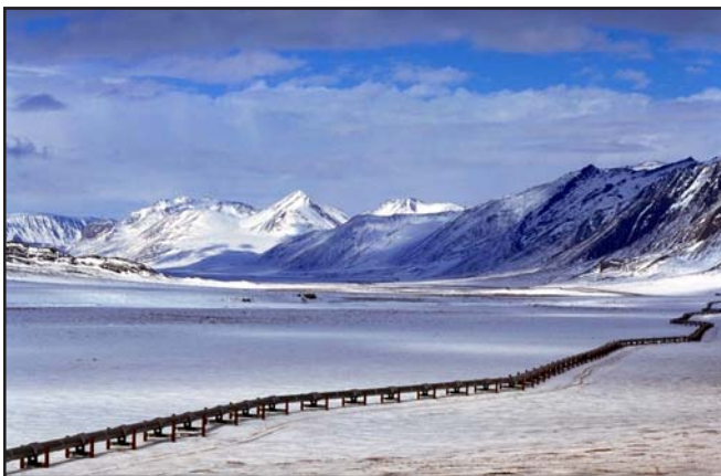
The 800-mile trans-Alaska pipeline currently transports nearly 1 million barrels per day of crude oil across the Alaskan wilderness to the port town of Valdez. Total throughput to date is over 14 billion barrels.
