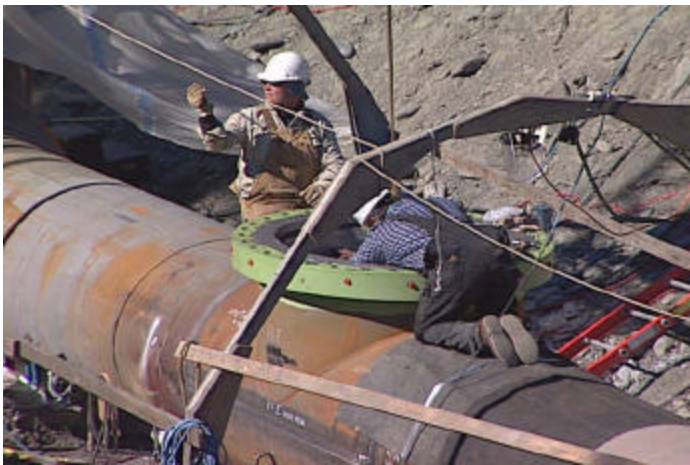
Figure 7: Split-Tee Assembly
