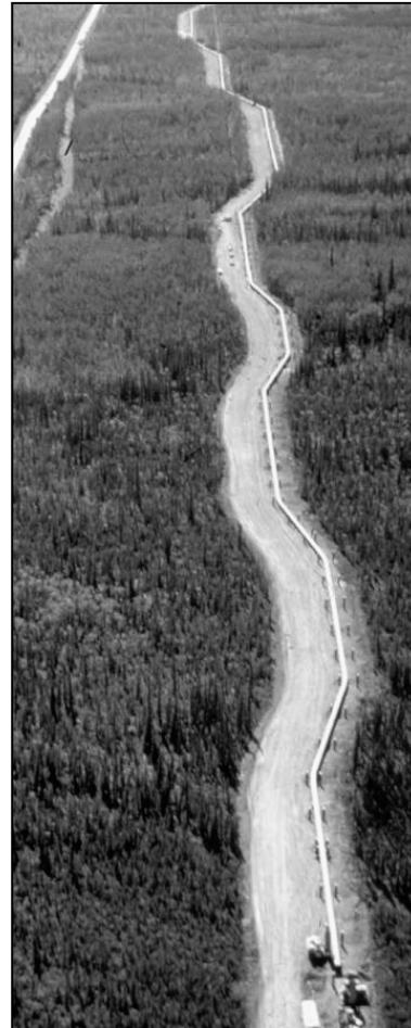
Figure 2. Trapezoidal or “zigzag” above-ground pipeline configuration.
