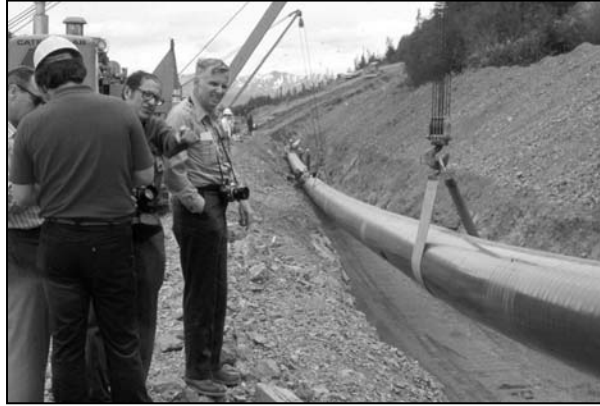
Figure 8. Buried TAPS pipeline section being lowered into trench during original construction in 1976.
