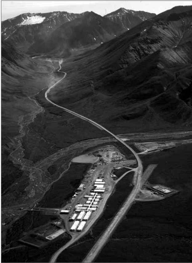
Atigun Construction Camp was one of 30 camps operating during pipeline construction. The buildings were removed and the site was revegetated in 1978.
