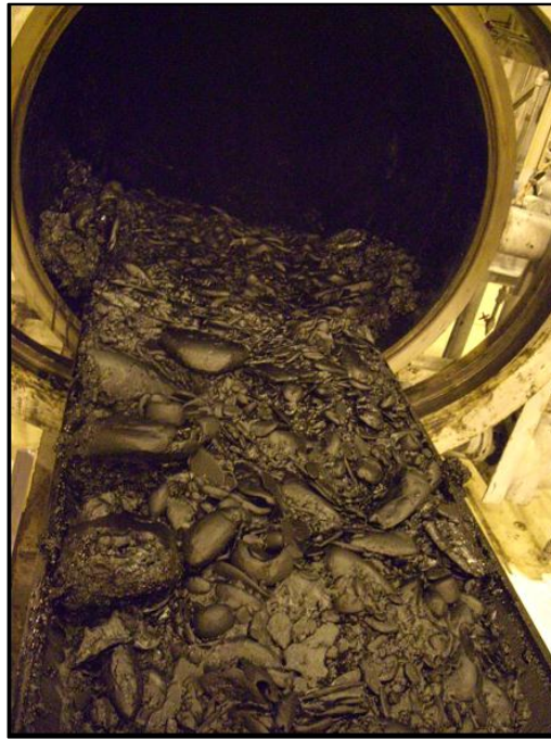
Figure 9. Pipeline Wax Removed from PS04 Pig Trap, March 2010
