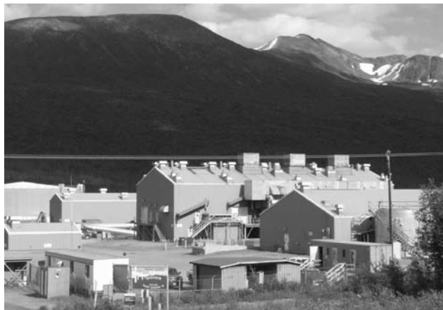
Pump Station 12, 65 miles north of Valdez, is in the southernmost station, pushing the oil up and over Thompson Pass.
