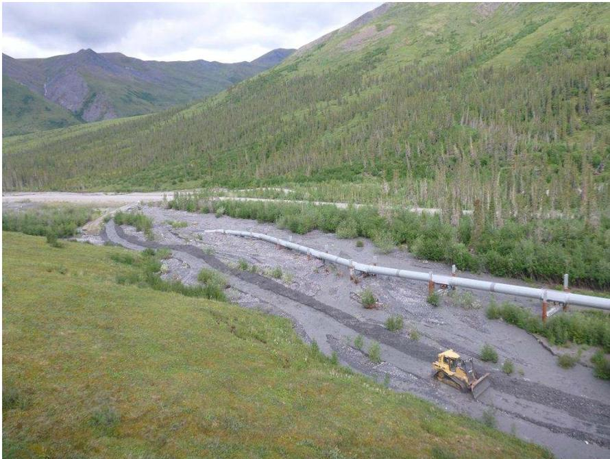
Excavator use was a luxury at the Beaver Brook flooding site, which is 32 miles south of Pump Station 4 at Milepost 176. A three-week-long July rainstorm on the Chandalar Shelf routed water and material downhill, turning the usually passive Beaver Brook into a raging, murky river. Phil Huelskoetter, a Pump Station 4 Baseline Foreman, said the silty material washed away the dike and engulfed the pipe like concrete.
