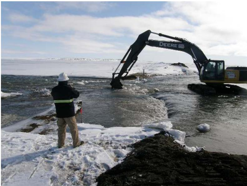
When the surging Sagavanirktok (Sag) River began carving away at underground pipeline coverage between Dalton Highway Mileposts 18-19 in May, TAPS employees responded. When a July rainstorm created a wild waterway that began encasing nearly 300 feet of aboveground pipe north of Pump Station 4 with quick-hardening shale, TAPS employees responded.
